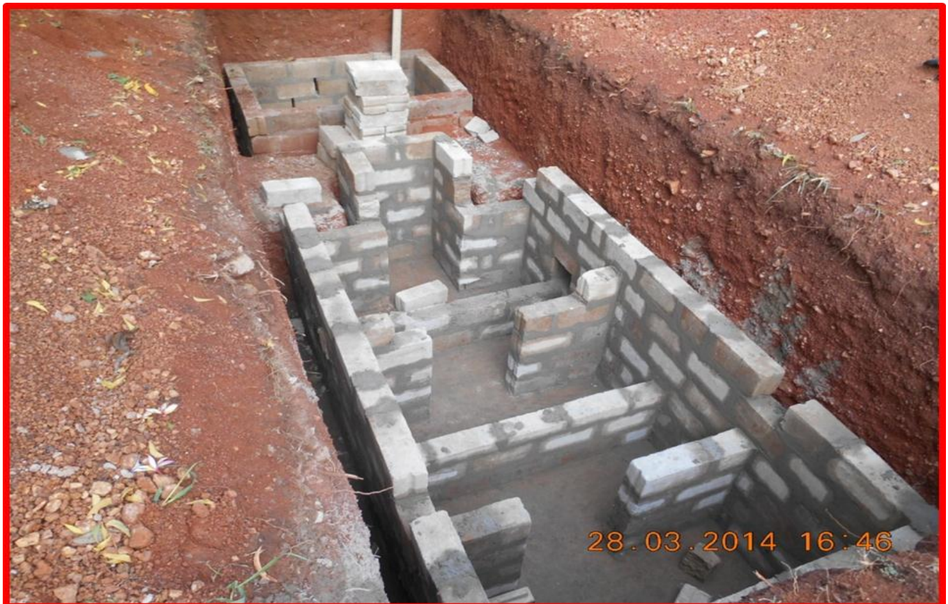
Figure 3: On-going construction of Anaerobic Baffled Bio-Digester showing concrete base and Baffles.
